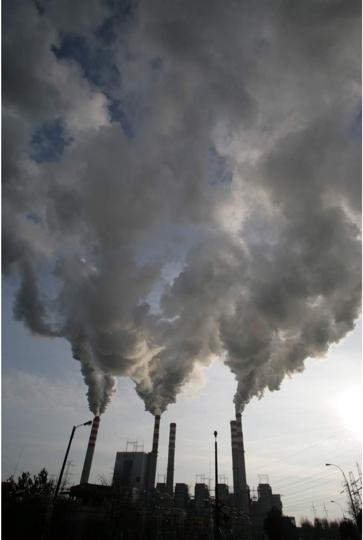
PGE's lignite-fired Belchatów plant is Europe's largest single point source of CO 2 emissions.
