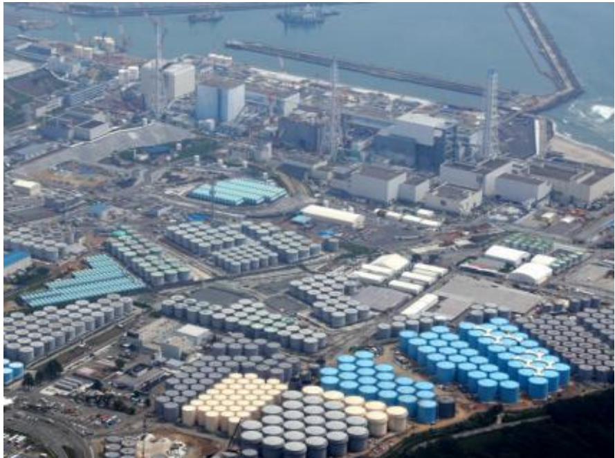
Wastewater storage tanks at Fukushima Daiichi NPP
