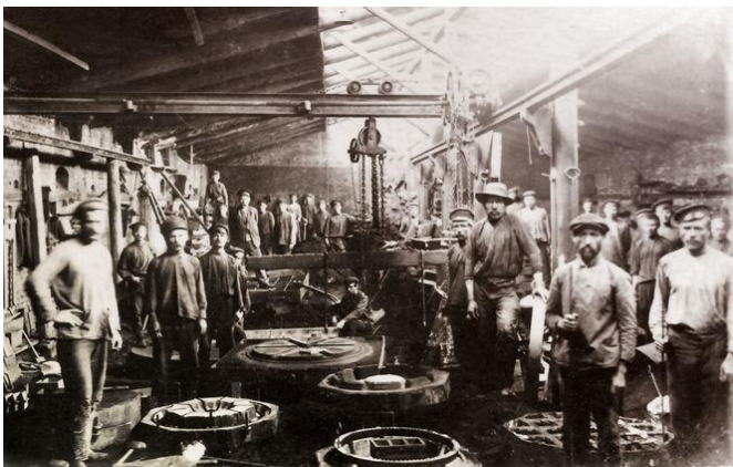
Donetsk in the early 1900s. Workers in the foundry of the agricultural machinery plant established by the American capitalist Jacob Niebuhr
